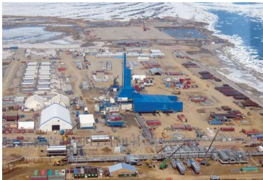
Fig. 1—Aerial view of Chayvo onshore well pad.
