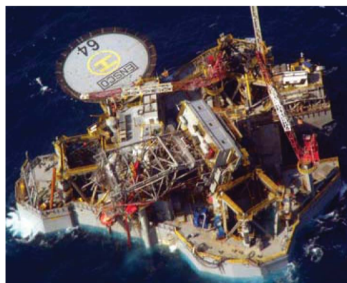
Fig. 1—Ensko 64 after Hurricane Ivan.
