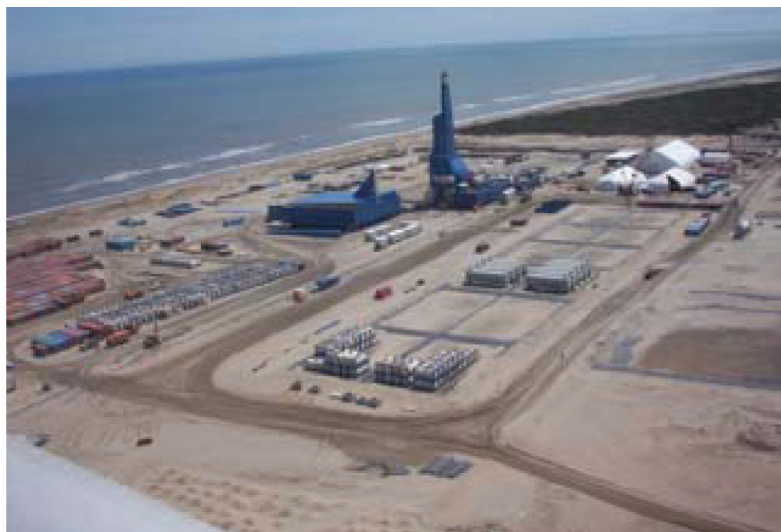
Fig. 1—Yastreb Rig 262 pipe barn during assembly.
