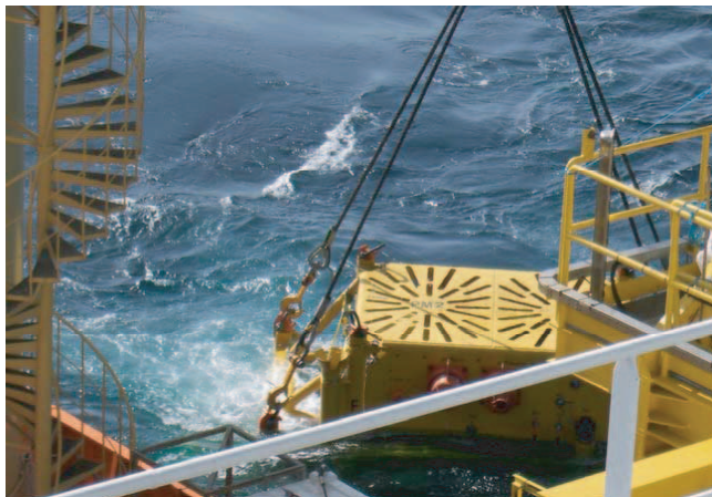
Fig. 2—(clockwise from top) Subsea configuration of the BP King field in the GOM, including addition of two multiphase boosting pumps, is shown. A pump is shown in closeup view and as it is being lowered into the water in 2007. The twin-screw, positive-displacement pumps are expected to increase the field production rate by 20% and total recovery by 7%. The pumps, in 5,600 ft of water, are the world’s deepest to date. Their tieback distance of 18 miles is the world’s longest for pumps. (Images courtesy of Aker Solutions.)
